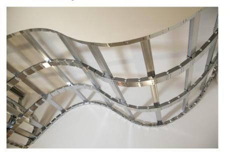
proceed with the plasterboard laying (thickness 6mm/10mm), that will find a continuous surface for optimum shaping
