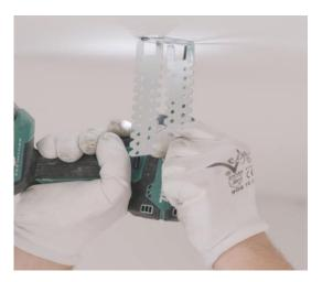
• Fix the standard studs on one side to the COBRA 30mm fixed to the lower side of the downstand, and on the other side to the universal brackets
