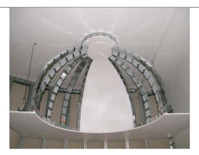
N.B.: If the dome is very big, it is necessary to place some more CONCAV / CONCAVEX Studs to strengthen the structure behind. Place them across the CONCAV / CONCAVEX already in place (double metal framework) and fix them behind the first ones with channel hangers.
