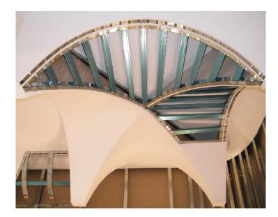
proceed with the plasterboard laying (thickness 6mm/10mm), that will find a continuous surface for optimum shaping.
