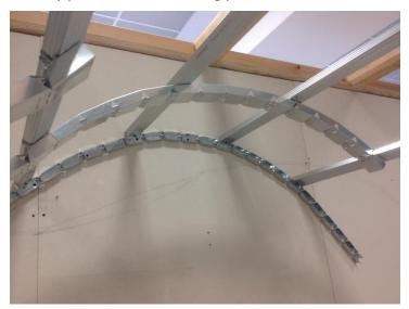
• connect the Studs with a channel connector 60x27 to obtain the curvature with the desired radius (if you are using the single CONCAVEX stud, no joint is necessary to change the direction of curvature, but only for the continuation beyond 3 metres)
