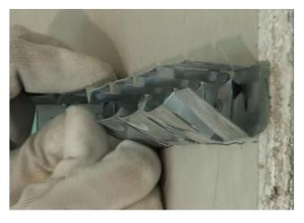
build the vault with a double metal framework: for the primary structure use C49x27 (or C60x27), for the secondary structure use the CONCAV / CONCAVEX Curving Stud and channel hangers (as for a flat ceiling)
