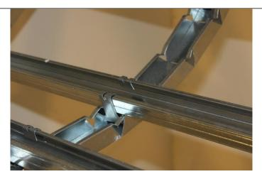
• the number of hangers and their positioning on the ceiling will be done accordingly to the size of the room and the additional loads
